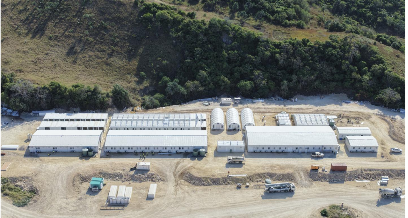
Image: Construction Camp and Kitchen areas of the Central Lime Project
